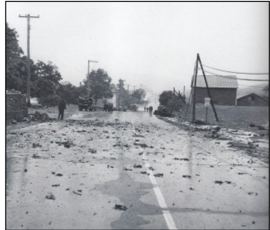
Debris strewn on Route 122 (Now Route 61) Photo © Pottsville Fire Department
