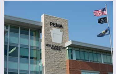
PEMA Headquarters, Harrisburg, PA
