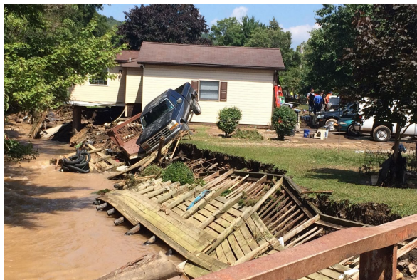
Storm damage in Connellsville, PA
